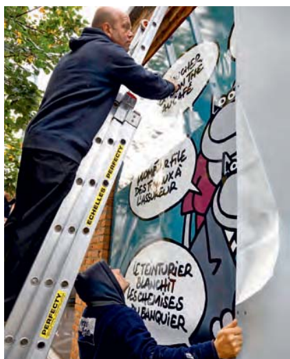
The adhesive films had to be applied to the panels on-site in order to ensure a seamless and hole-free visual.
